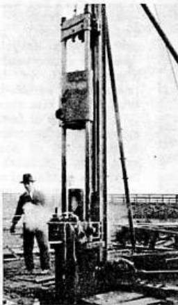
The Model D3 diesel pile-driver of 1937. The need for precision manufacture is indicated by the exposed, vertical piston, seen at the base of the guide bars along which, with the open cylinder formed in it, the 610kg hammer is descending.
