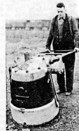
Soon after the end of World War Two this massive 508 and 1,016kg "Frog" rammer (so called because of its leaping forward motion) made its appearance.
