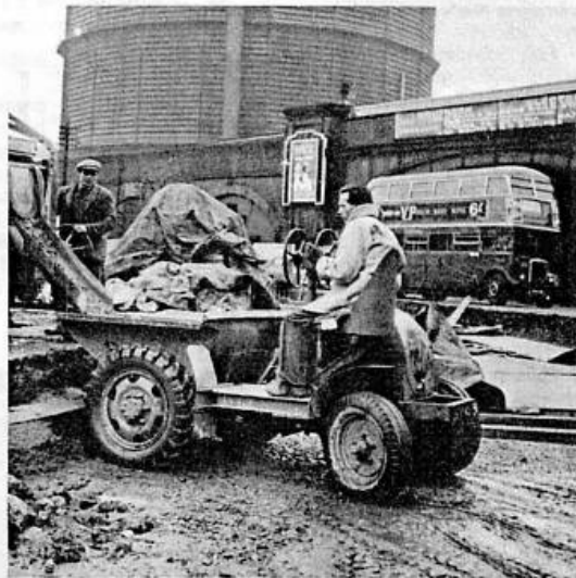
With reversible seat and twin steering wheels, this early Johnson site dumper, with one of the first small Petters diesels, is seen at work on the 1951 Festival of Britain construction in South London.
