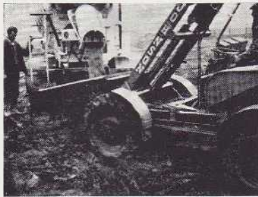
The Humber can be fed by a mixer or ready-mixed transporter.
